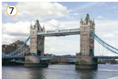
Tower B ridge
